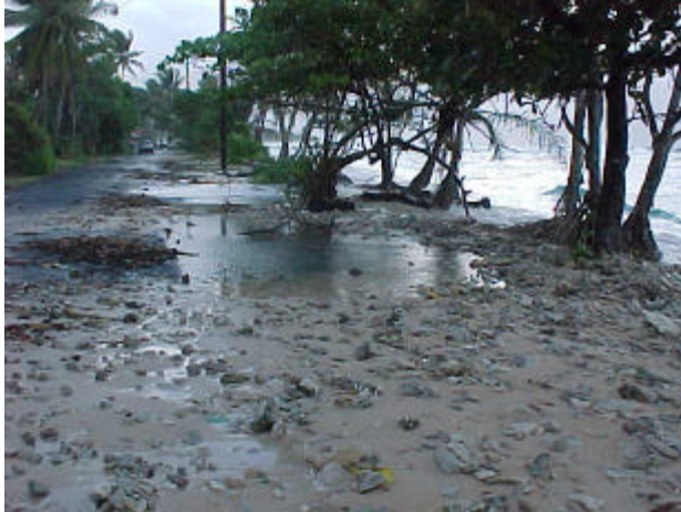
Figure 10 Storm damage to the road at Kotfwa in Malem
