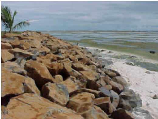
Figure 14 The rock revetment at Finaunpes
