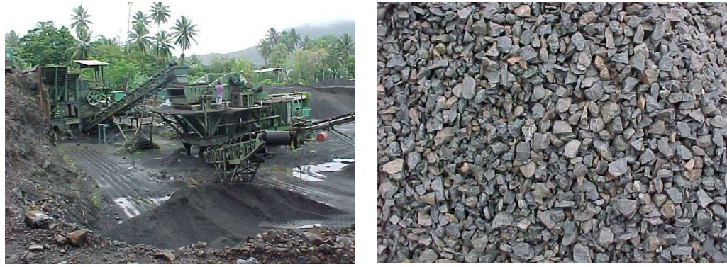
Figure 12: The crushing plant and quarry at Sansrick, and the 1/2” chips produced.
